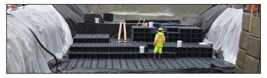
The expert team at GRAF & BARR Plastics Inc specified, designed and supervised the installation of three stormwater infiltration systems, which were fitted in two phases. During the first phase, a 1,180 m³ two-tank system was installed. It was built using 5,760 heavy-duty EcoBloc Inspect Flex modules to meet a burial depth of 5 meters with in-built inspection channels for easy maintenance. During phase two, a second, 658 m³ system was fitted consisting of 3,210 EcoBloc Inspect Flex modules.
